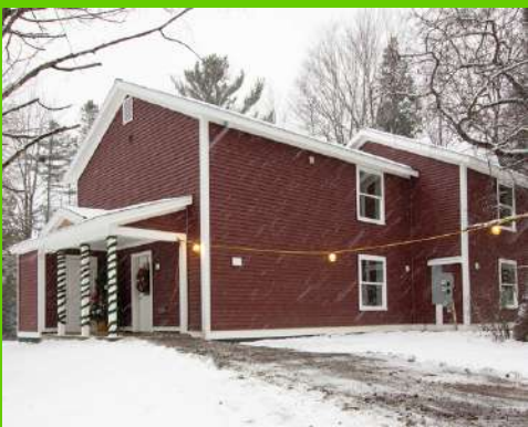
One of the newly-renovated duplexes at Burkeland Lane.
