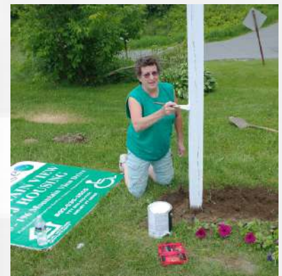
RuralEdge resident Mary Brown paints the posts before helping install the new property sign at Mountain View Housing in St. Johnsbury..
